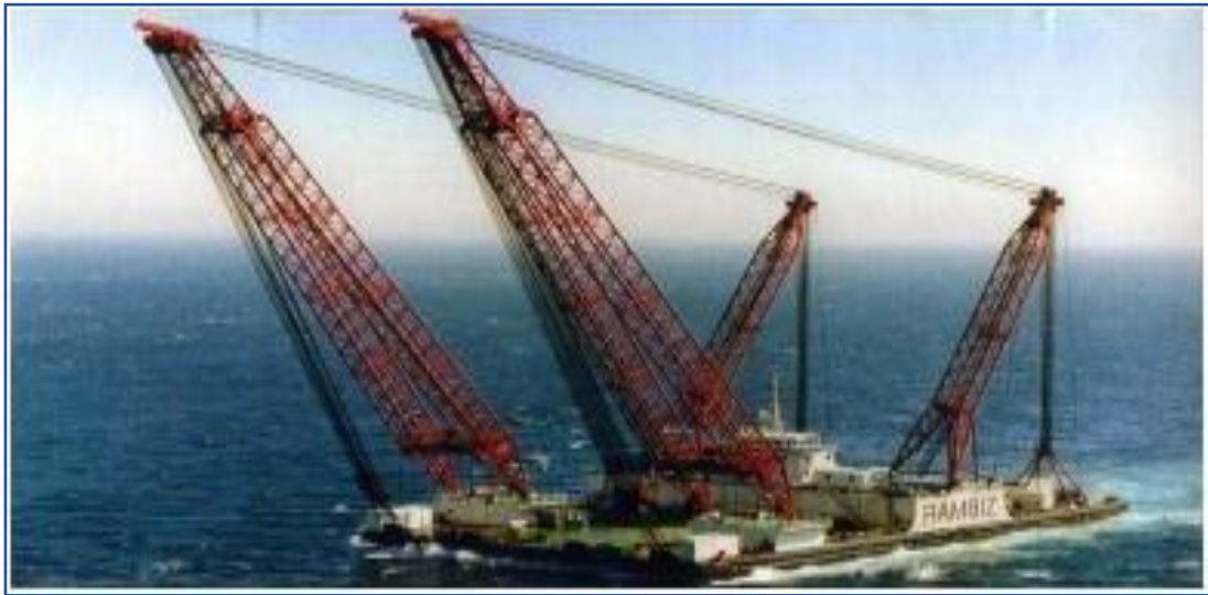
Figure : I-11 :Grues Flottantes
