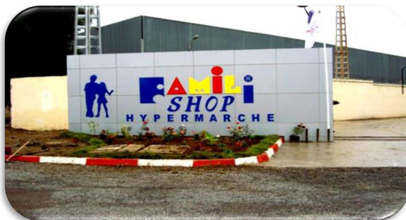
Figure 3.4 : La façade de Famili Shop Blida
