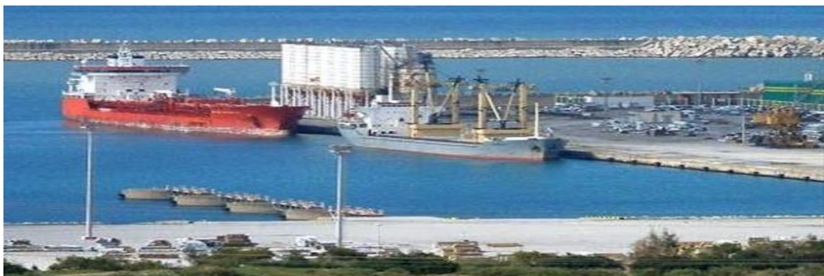
Figure 5.13 Port of Djendjen Algeria: The Custom Free Port
